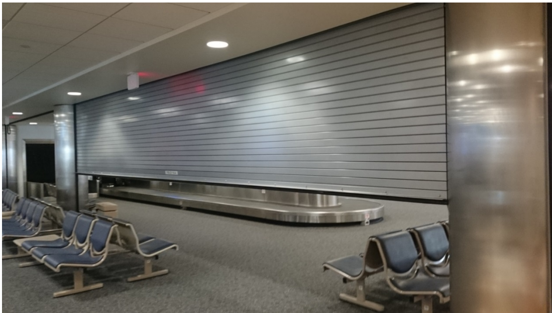
Figure 5-9: Partition Lowering to Enable a Baggage Carousel to be Used for International Flights
