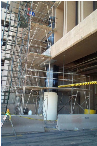
Figure B-4. Wrapping Process—Kevlar-Carbon Fiber Wrap
