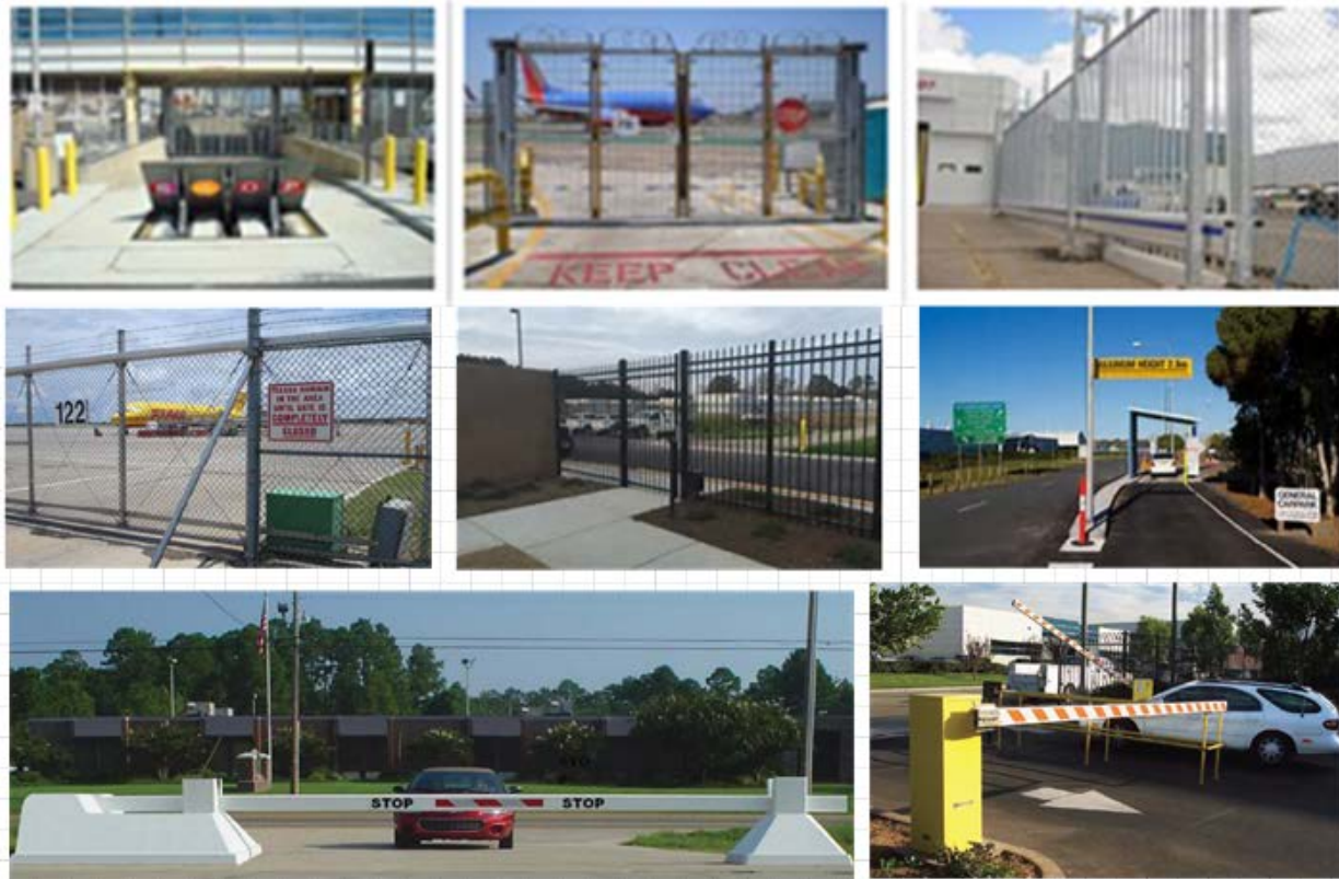
Figure 11-2. Examples of Airport Gate Installations
