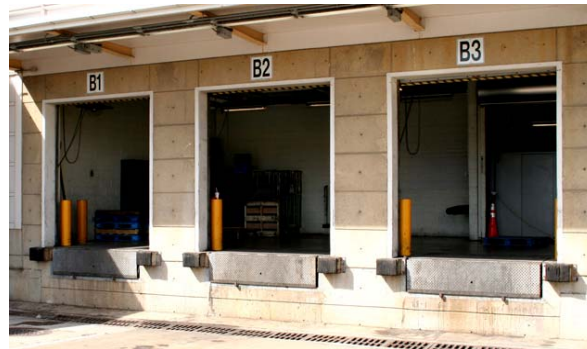
Figure B-6. Loading Dock
