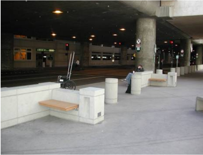
Figure B-14. Vehicle Barrier—at Grade
