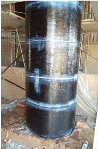
Figure B-11. Column Wrapping Procedure
