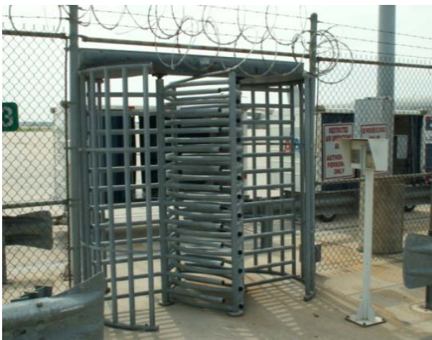
Figure 7-3. One-Way Revolving Personnel Gate
