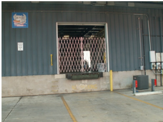
Figure 7-1. Scissor Gate on Public Side of Building
