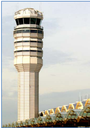
Figure B-8. ATC Tower
