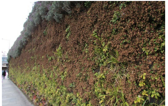
Figure A-1. Example of CPTED: a wall designed to prevent graffiti
