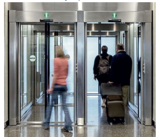
Figure 11. Example of Lights Used to Identify Open Lanes
