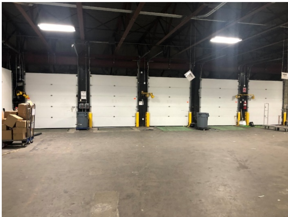
Figure B-9. Case Study 1: Distribution Doors from Interior
