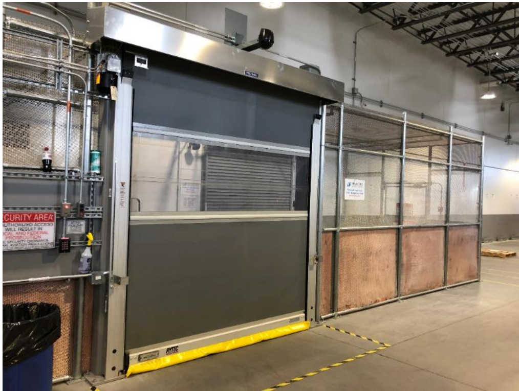
Figure B-28. Case Study 3: Warehouse Looking at Screening Portal
