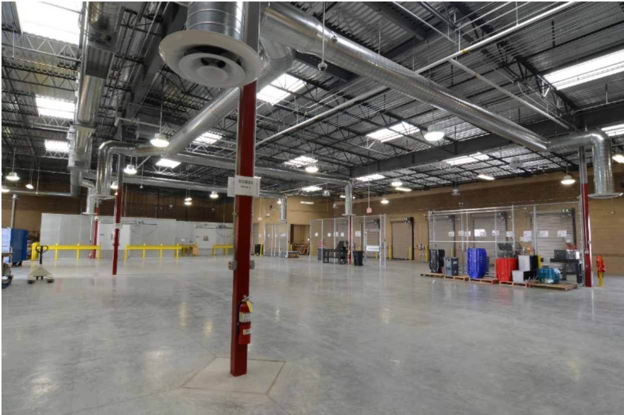
Figure B-48. Case Study 5: Interior Secure Warehouse
