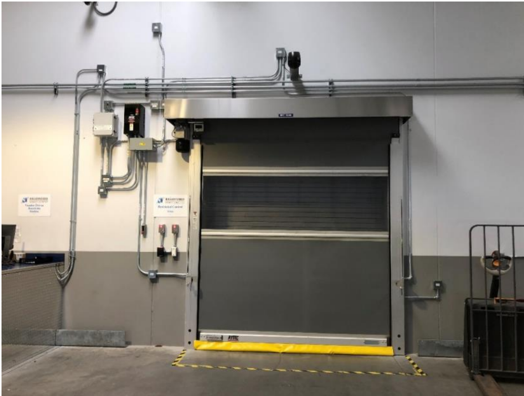
Figure B-27. Case Study 3: Receiving Looking at Portal
