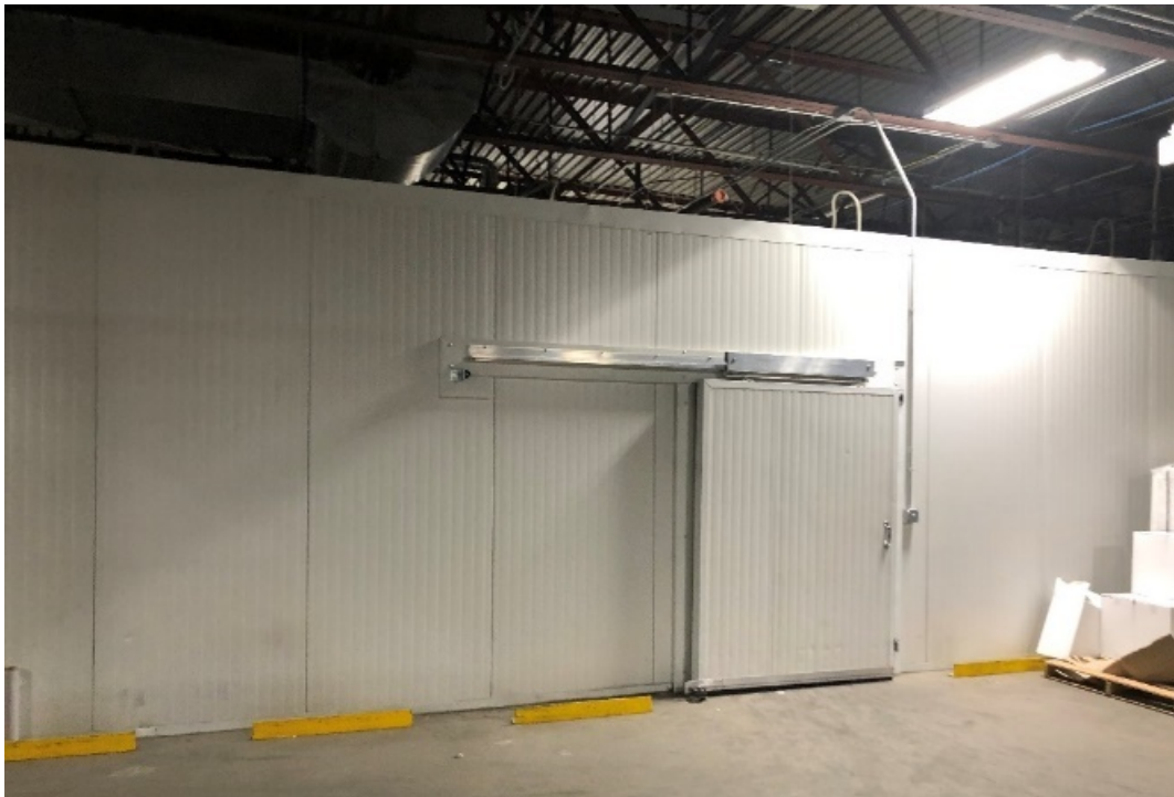
Figure B-7. Case Study 1: Cooler and Freezer in Warehouse
