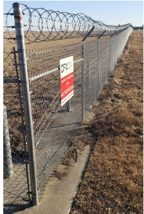
Figure 11. Sample Airport Perimeter Fence
