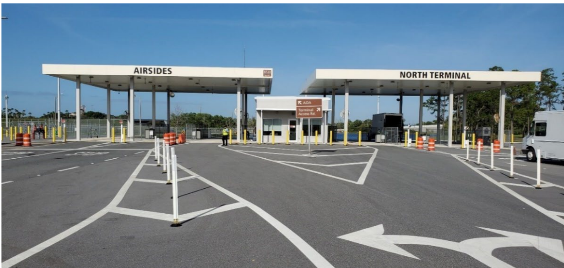
Figure F-2. Gate Approach Area
