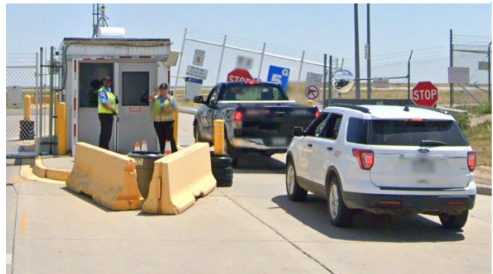
Figure 3-3. Pivot Gate at a CAT X Airport
