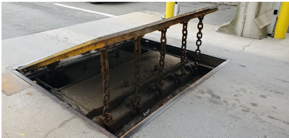
Figure D-12. Hydraulic Wedge Barrier in Deployed Position
