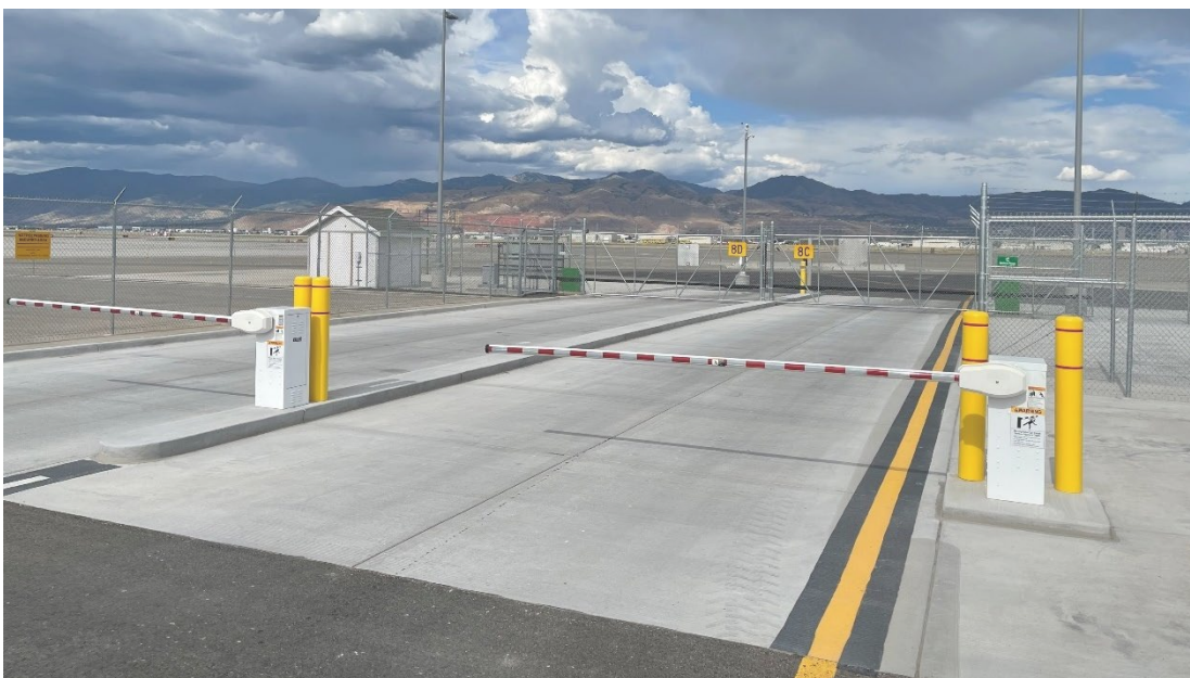
Figure 2-3. Sally Port at a CAT X Airport
