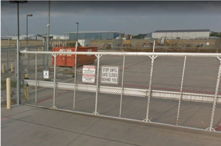
Figure 3-2. Cantilever Gate at a CAT I Airport
