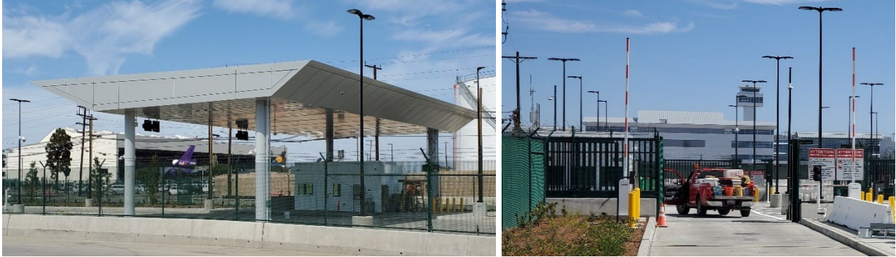
Figure E-1. New Vehicle Access Gate During Construction
