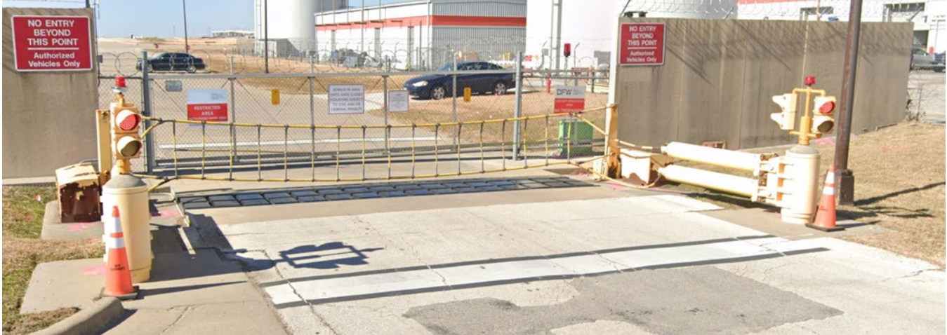
Figure 3-7. Net Barrier at a CAT X Airport
