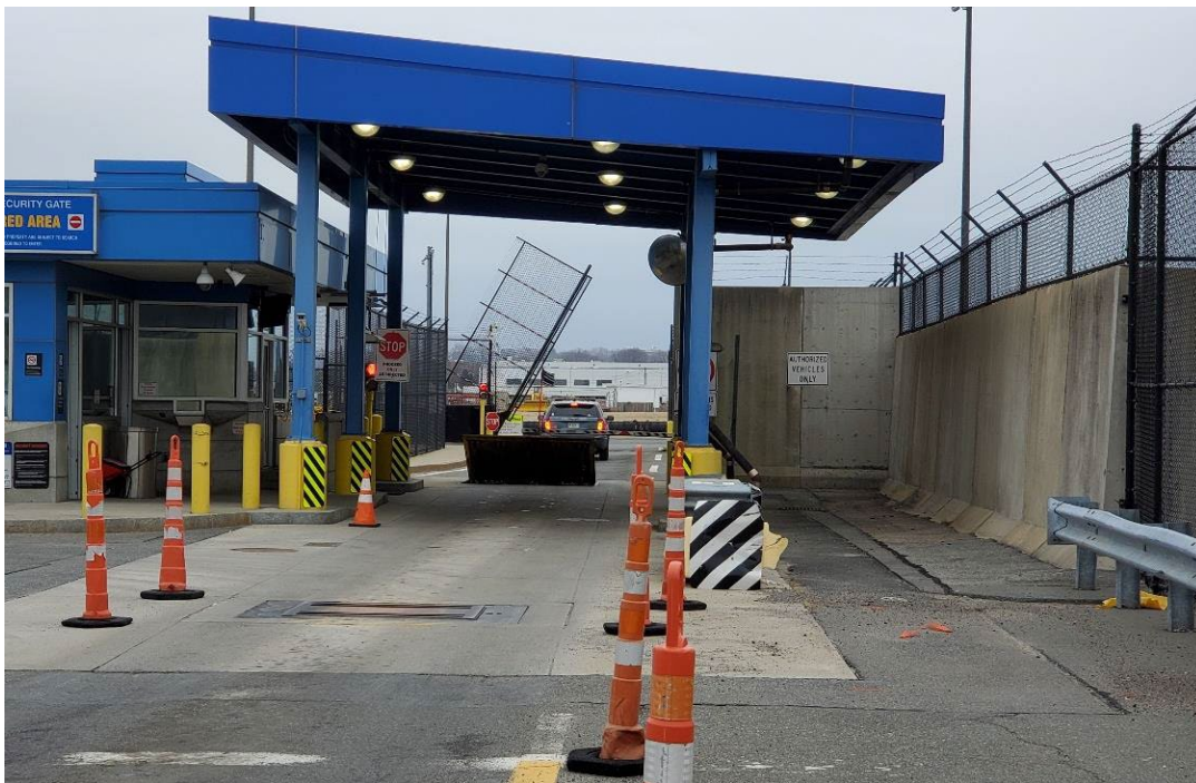
Figure D-2. Gate B Overview
