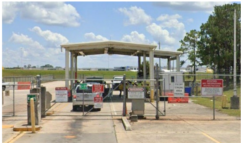
Figure 2-4. Overhead Covering at a CAT X Airport
