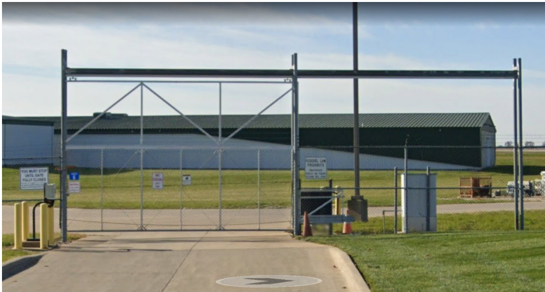
Figure 3-1. Overhead Sliding Gate at a CAT II Airport
