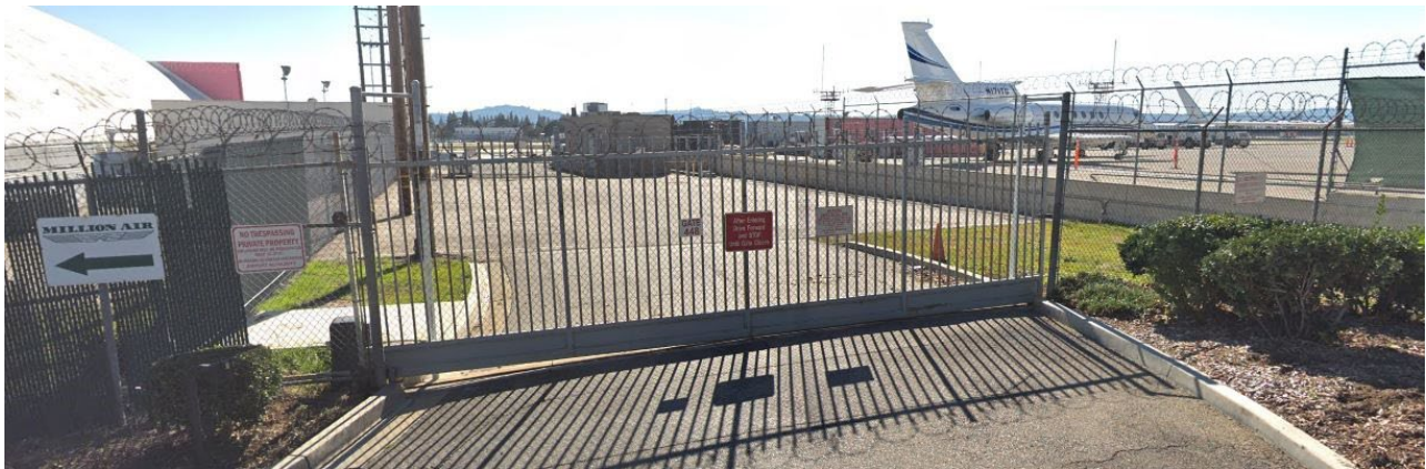
Figure 3-8. Vertical Bars on a Gate at a CAT I Airport
