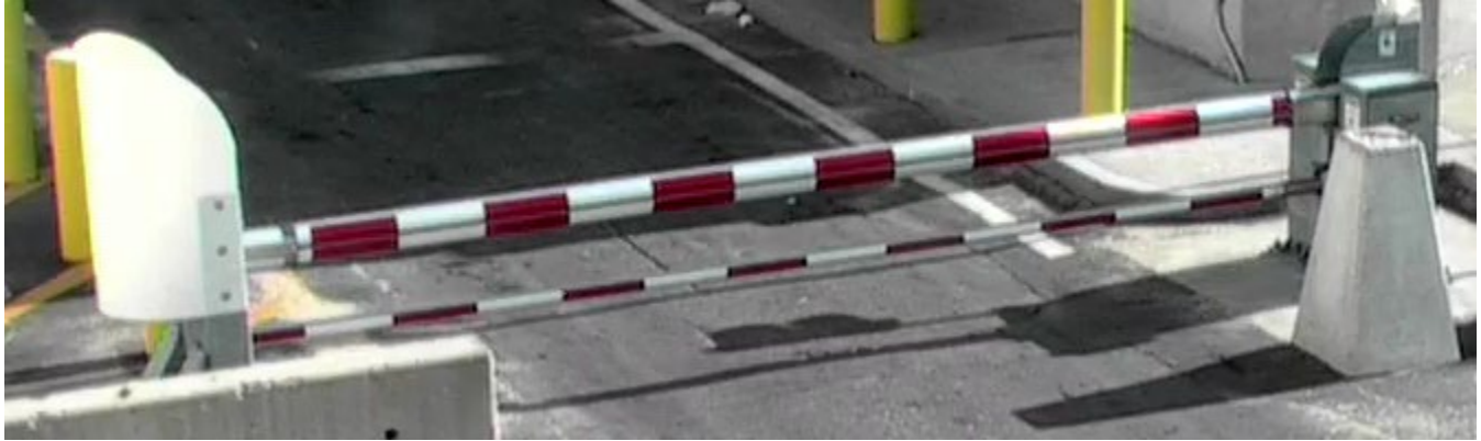
Figure D-10. Crash-Rated Arm Barrier, Lowered and Locked
