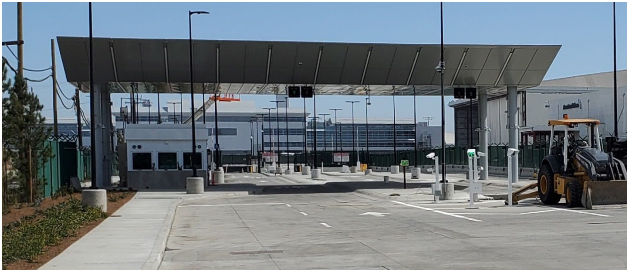
Figure E-2. Shelter with Integrated LED Lighting Strips
