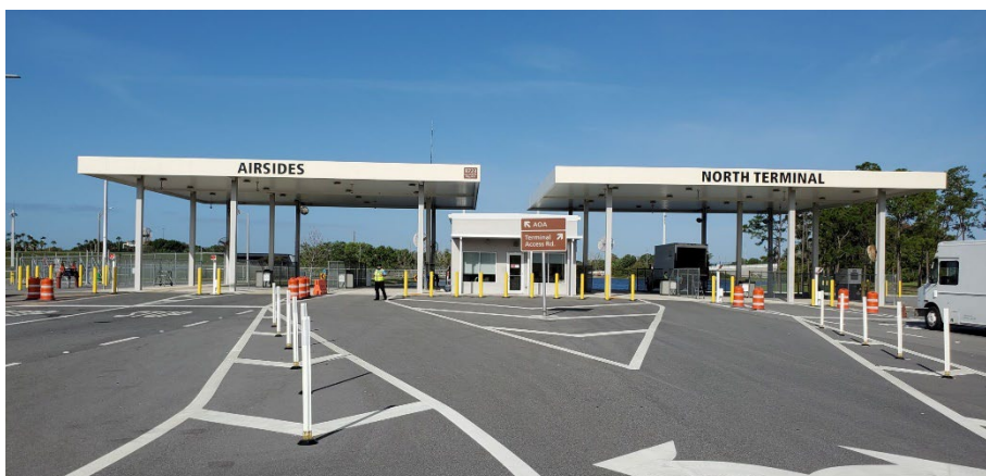
Figure 4-5. Common Traffic Markings at a CAT X Airport
