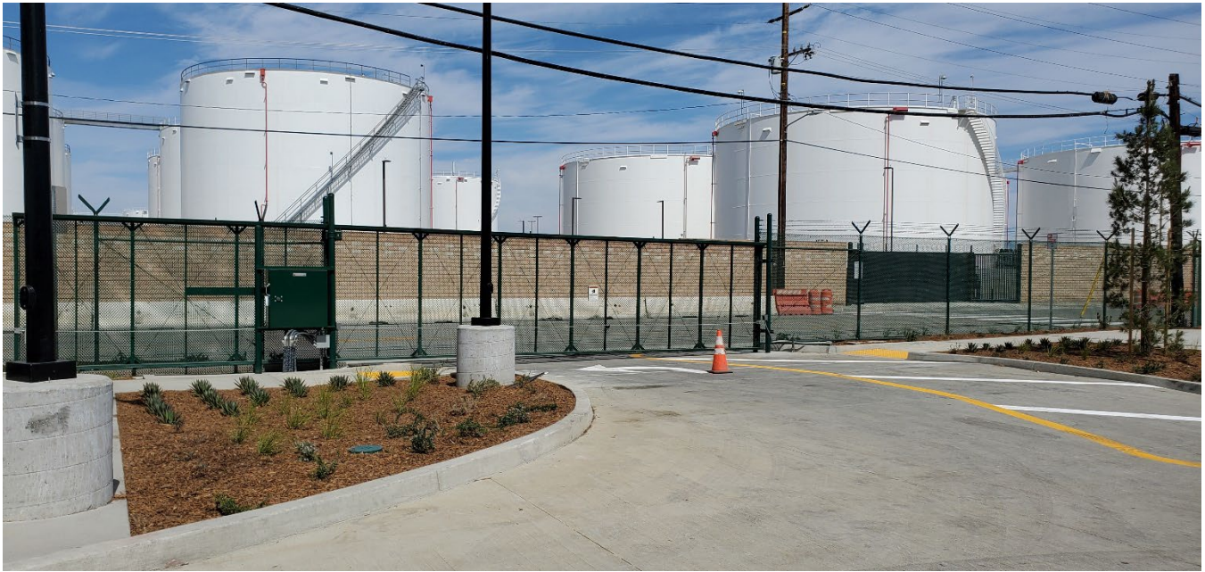
Figure E-3. Vehicle Reject Gate
