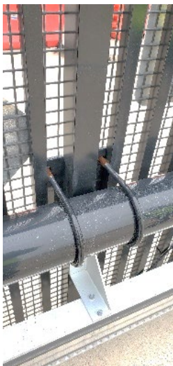
Figure A-4. Attachment via U-Bolts
