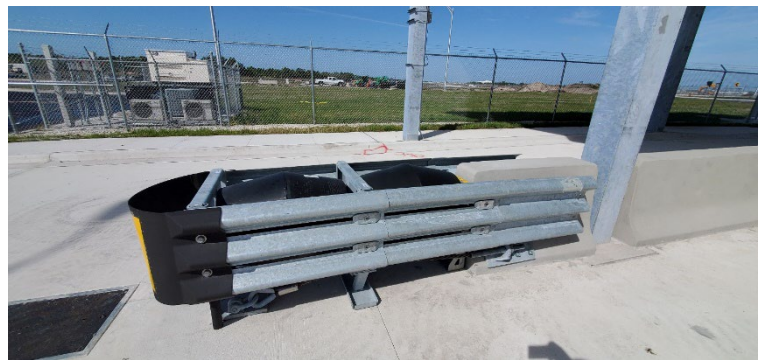
Figure F-4. Sacrificial Energy-Absorbing Crash Protection
