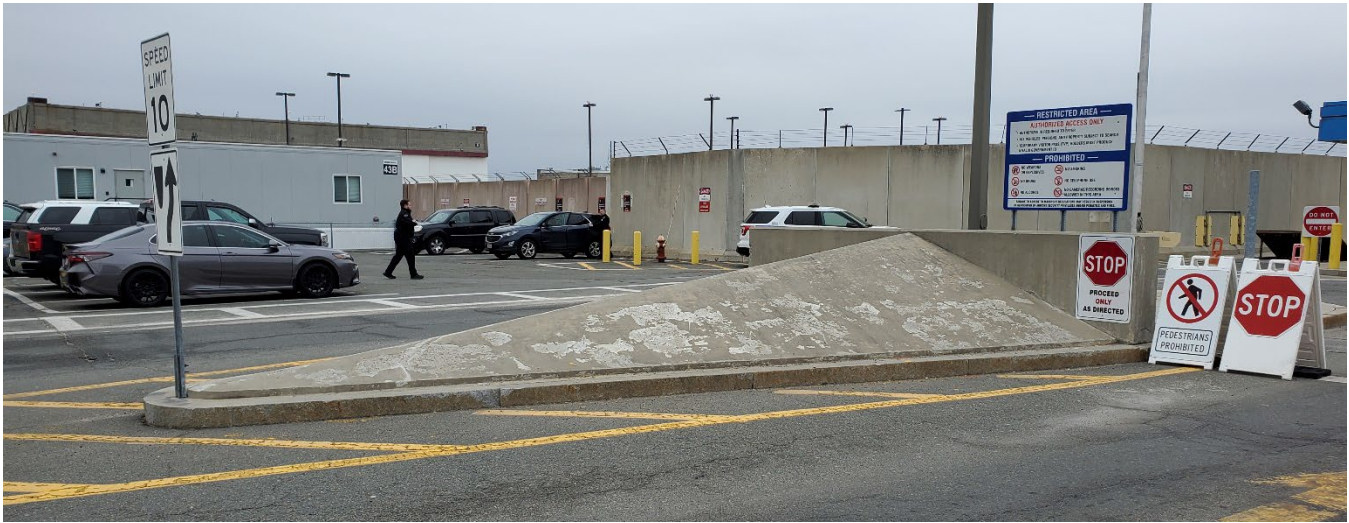
Figure D-5. Concrete Vehicle Diverter
