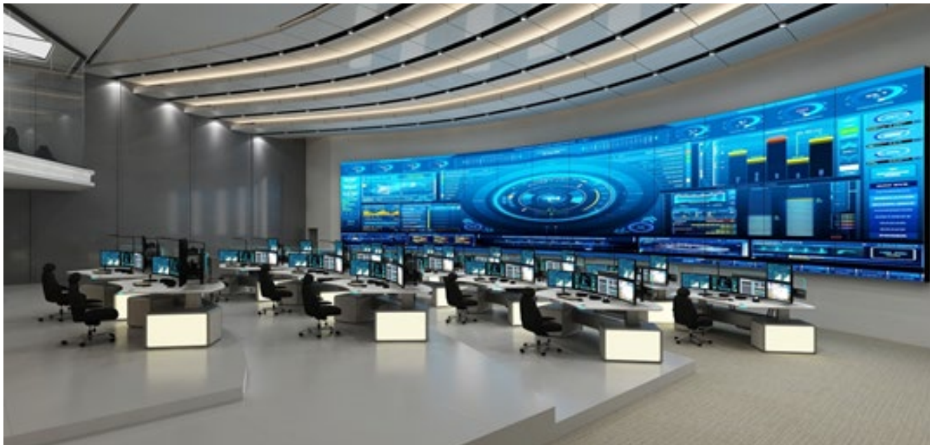
Figure 4-1. Direct View LED Video Wall
