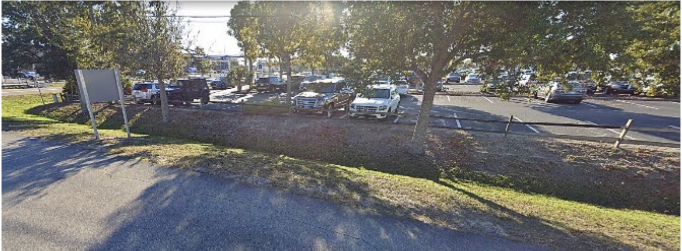
Figure 8-2. Example of a Drainage Swale Along a Parking Lot
