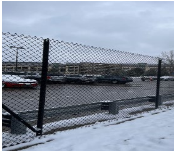
Figure A-16. Perimeter Fencing
