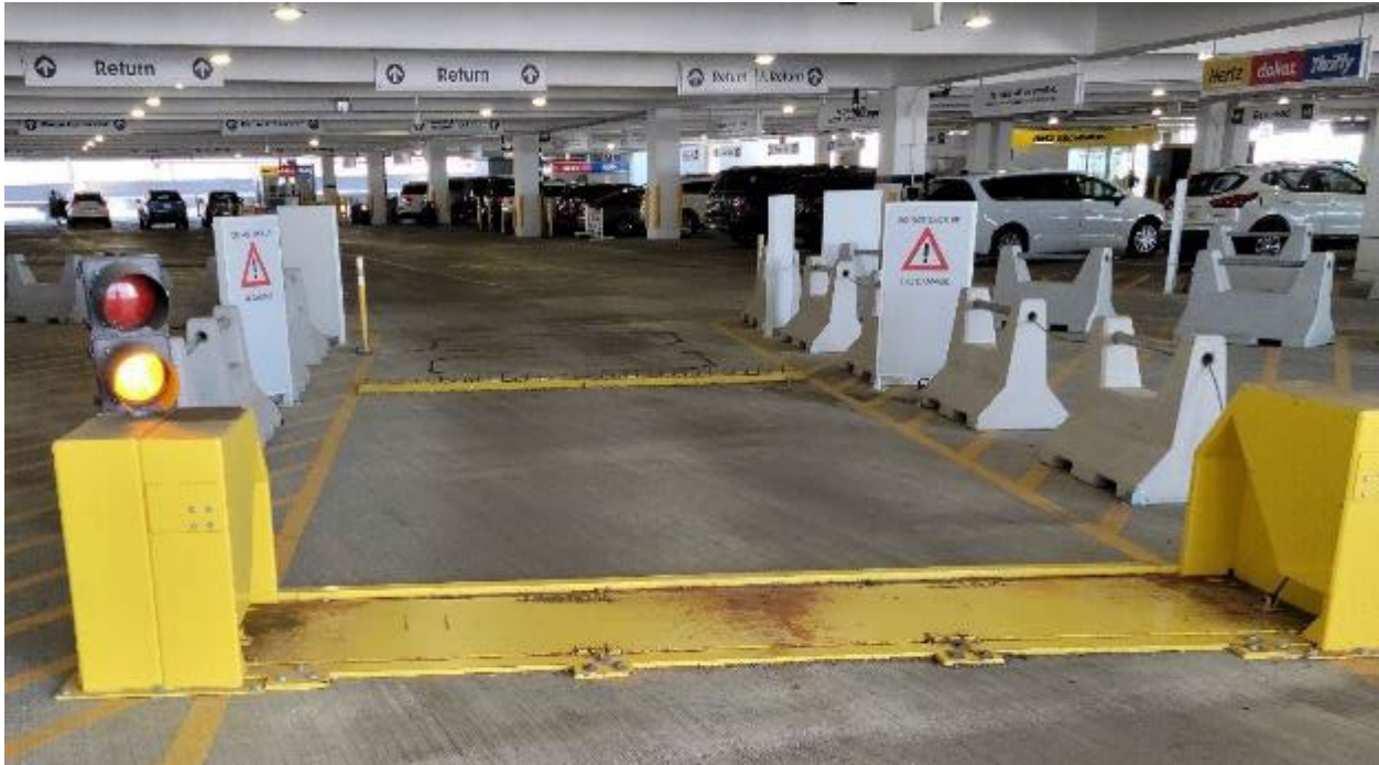
Figure A-11. Entrance with Double Barriers
