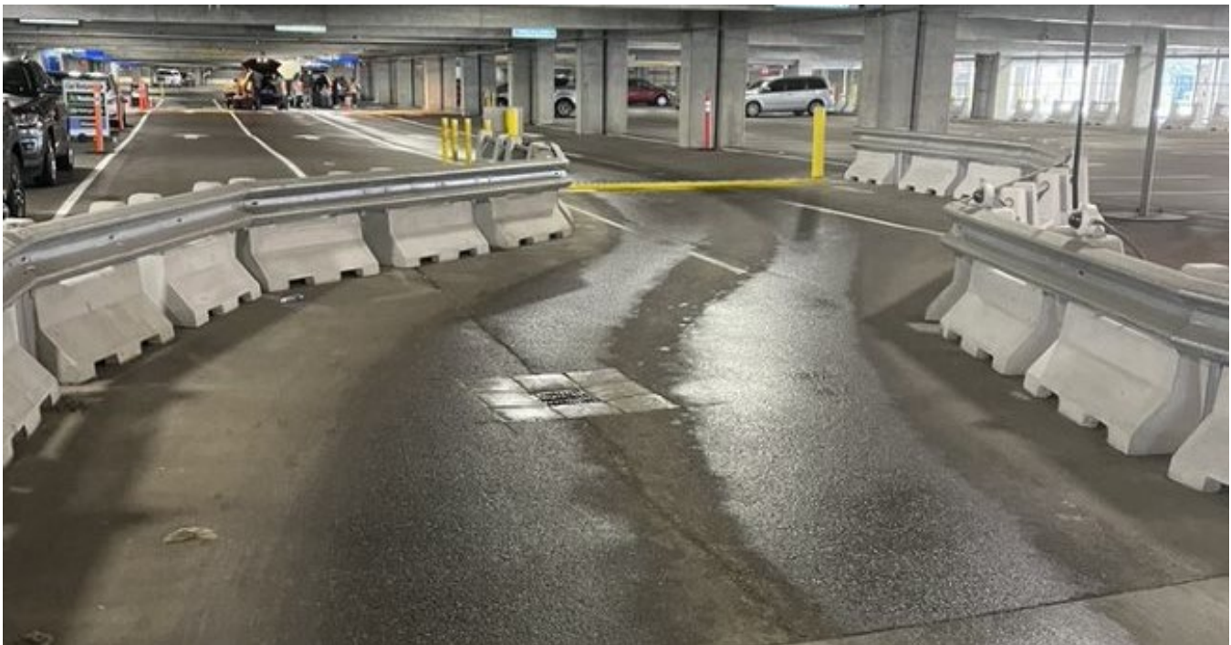
Figure 8-3. Concrete Barriers Delineating RAC Operators
