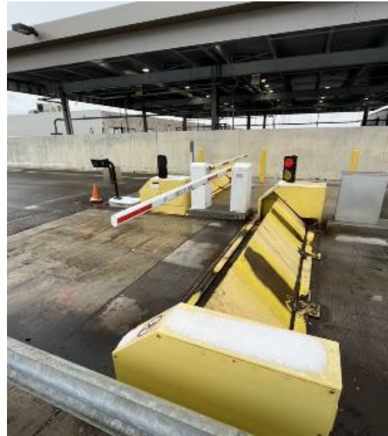
Figure A-15. Physical Access Control at Egress Portals
