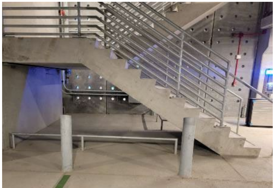
Figure 8-4. Open Sightlines in Stairwell to Reduce Concealment
