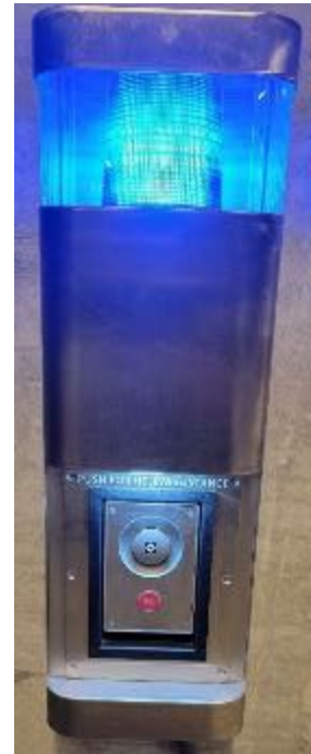
Figure 6-6. Example of a Duress Button
