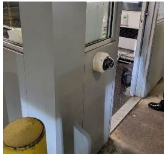
Figure 6-3. LPR Pointed at Vehicle Exit
