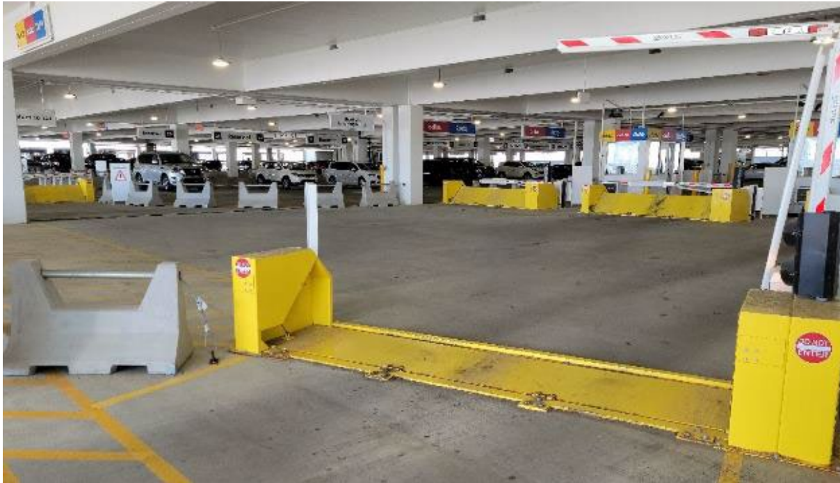
Figure A-13. Sally Port Exit
