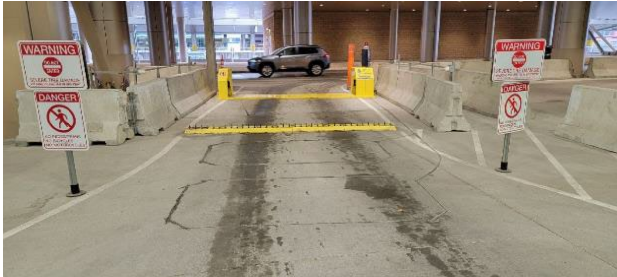
Figure A-3. Traffic Spikes and Plate Barrier at SLC RAC facility Entrance
