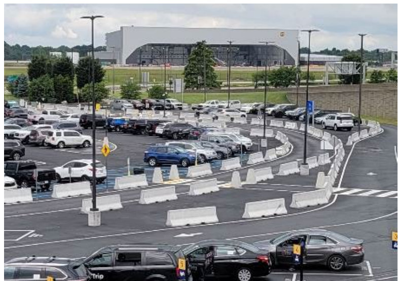
Figure 8-7. Traffic Calming Curved Lanes
