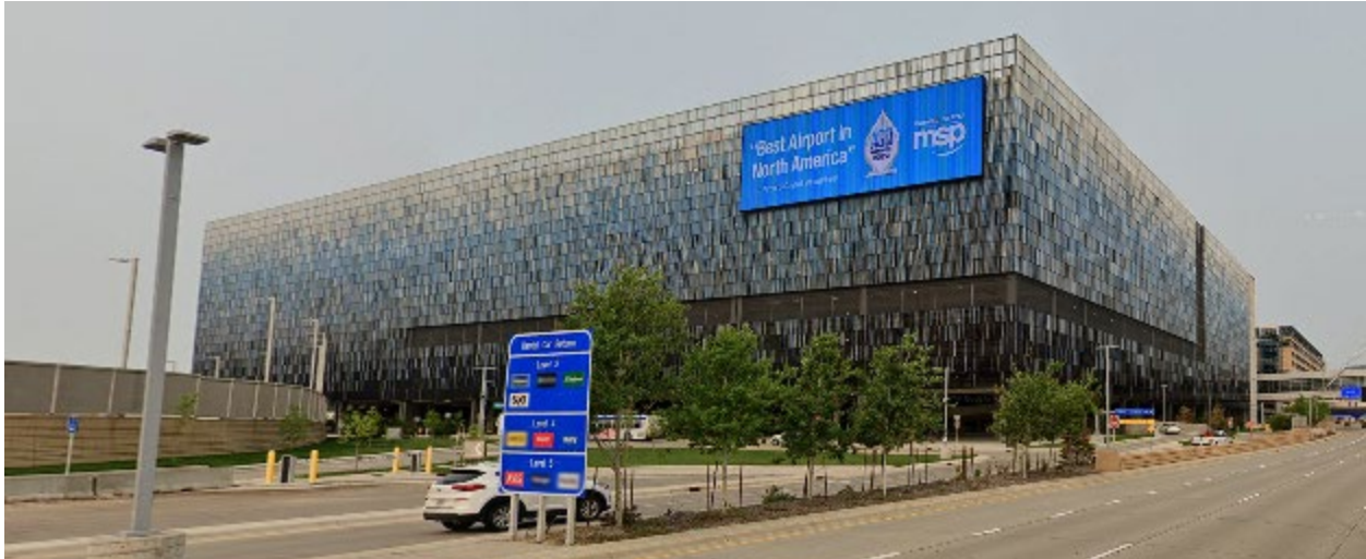
Figure A-20. T1 Silver Ramp Facility
