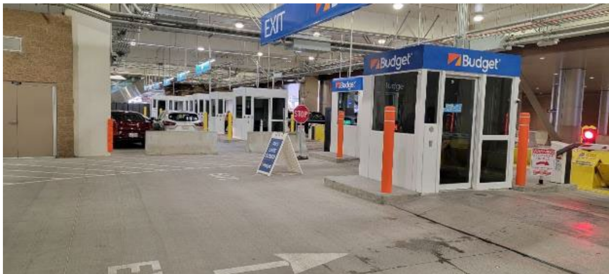
Figure A-2. Identical Security Booths and Barriers at All Exits
