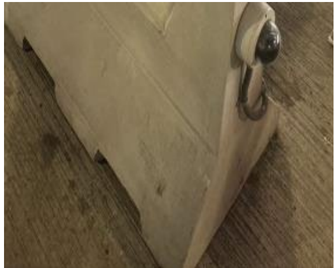
Figure A-22. Concrete Barrier with License Plate Camera
