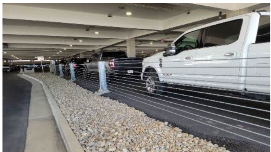
Figure A-10. Vehicle-Arresting Cable Perimeter
