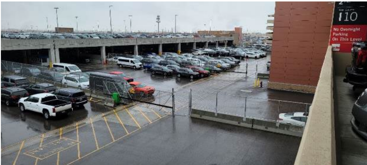
Figure A-5. Fire Lane in Fencing
