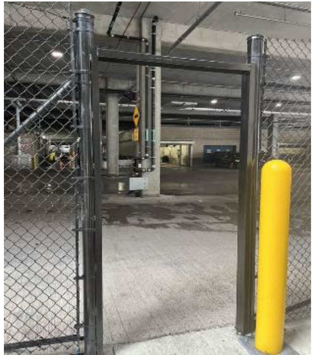
Figure A-27. Fence Prepped for Full Height Pedestrian Turnstile
