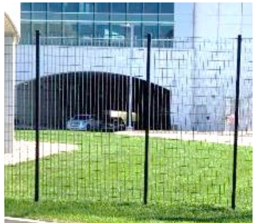
Figure 8-14. Example of Anti-Climb and Anti-Ram Fencing
