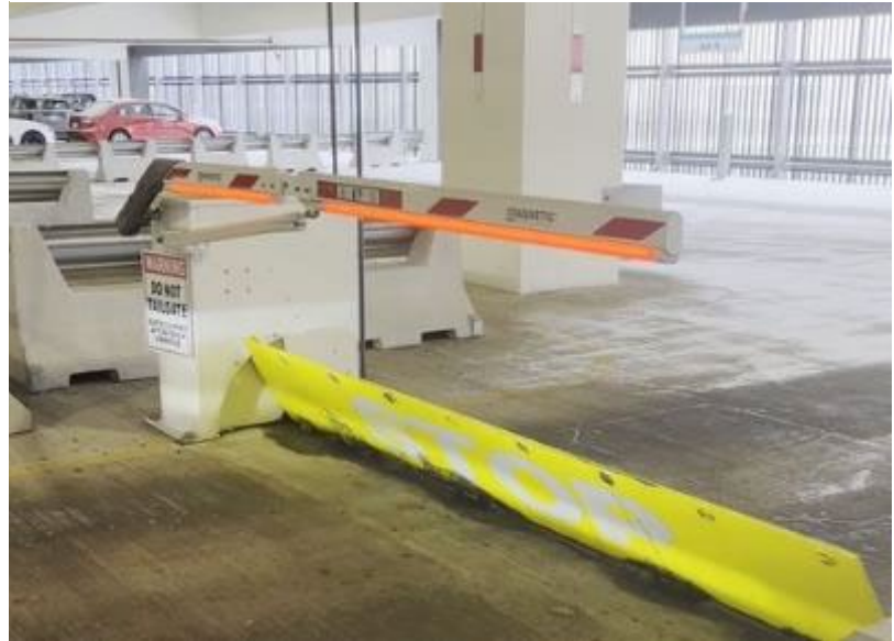
Figure 8-10. Example of a Plate Barrier and Barrier Arm
