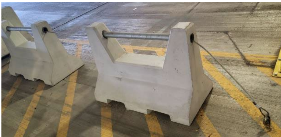
Figure 8-11. Concrete Barrier Attached to the Pavement and Anchored to Other Concrete Barriers
