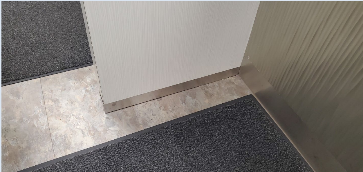
Figure 4-19. Metal Wall Protectors Around Workstations
