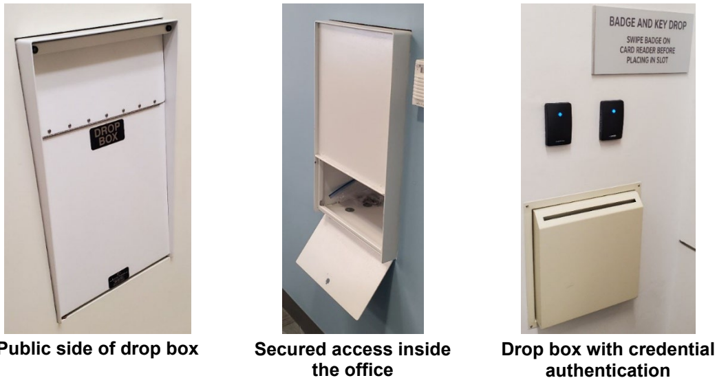
Figure 4-27. Secured Drop Box
